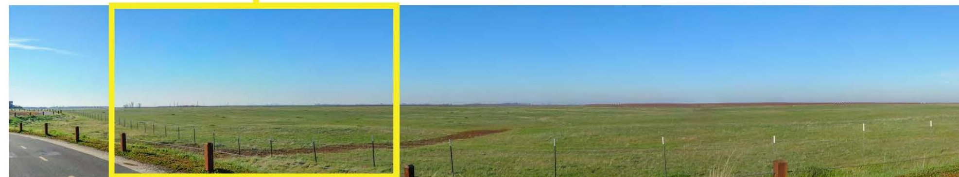
Exhibit 3.1-12. Viewpoint 3c Simulated Conditions Looking Southwest towards BESS Storage, Substation and Solar Facilities
